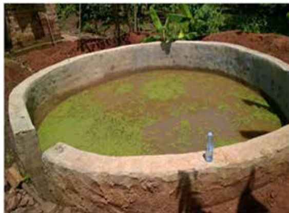
Figure 1. Water harvesting tank
